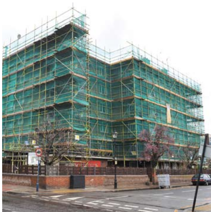
External work at Hooke House
