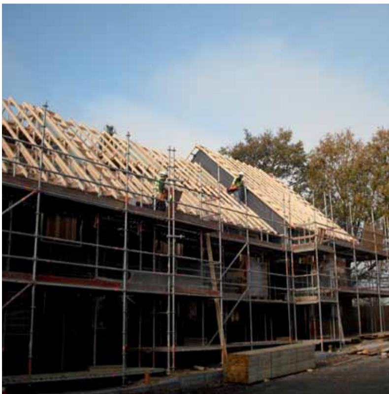
Construction work is well underway at Laundry Way.
