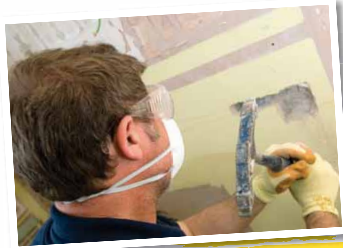
Terry from Wherry Maintenance Services working on a bathroom upgrad
