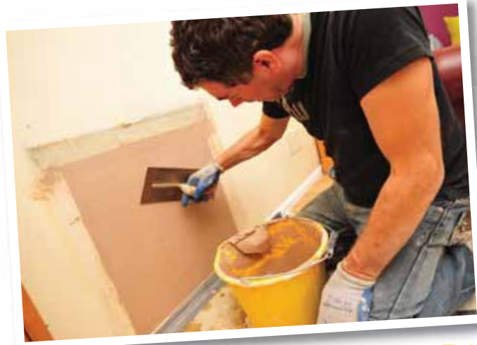
Adustus workman plastering the wall after removing an old gas fire
