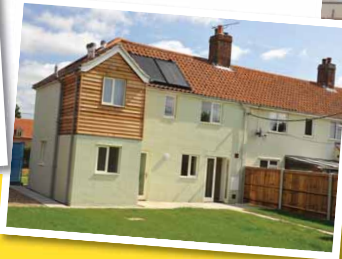
In progress of fitting external wall insulation to one of the homes in Crostwick, Norfolk
